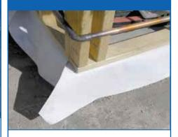
**HomeGuard DPC** (Damp Proof Course) is a tough 500 micron UV stabilised polymer sheeting containing Biflex Termiticide that offers both perimeter subterranean termite protection and damp proofing in one installation.
