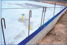
**HomeGuard PB** is manufactured from 300 micron, UV stabilized white polymer sheeting containing HomeGuard Termiticide which provides perimeter subterranean termite protection. This material is not rated to provide a damp proof course.
